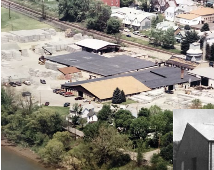
The Bauer Company manufacturing facility in Kittanning, PA in 1992. This facility was in operation from 1922 to 2003.
