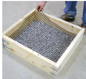
Geo-grid is added between layers of gravel.
