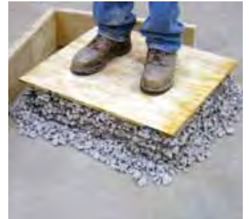
Geo-grid is added between layers of gravel.
